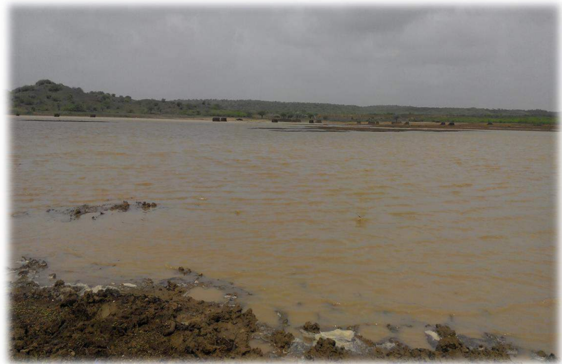
Dam preparation at Mata-No-Madh village
