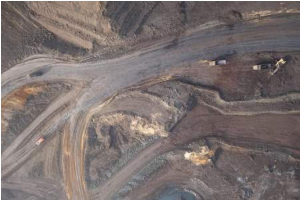
Fig 3.3.11 Aerial View of Material Transport Route
