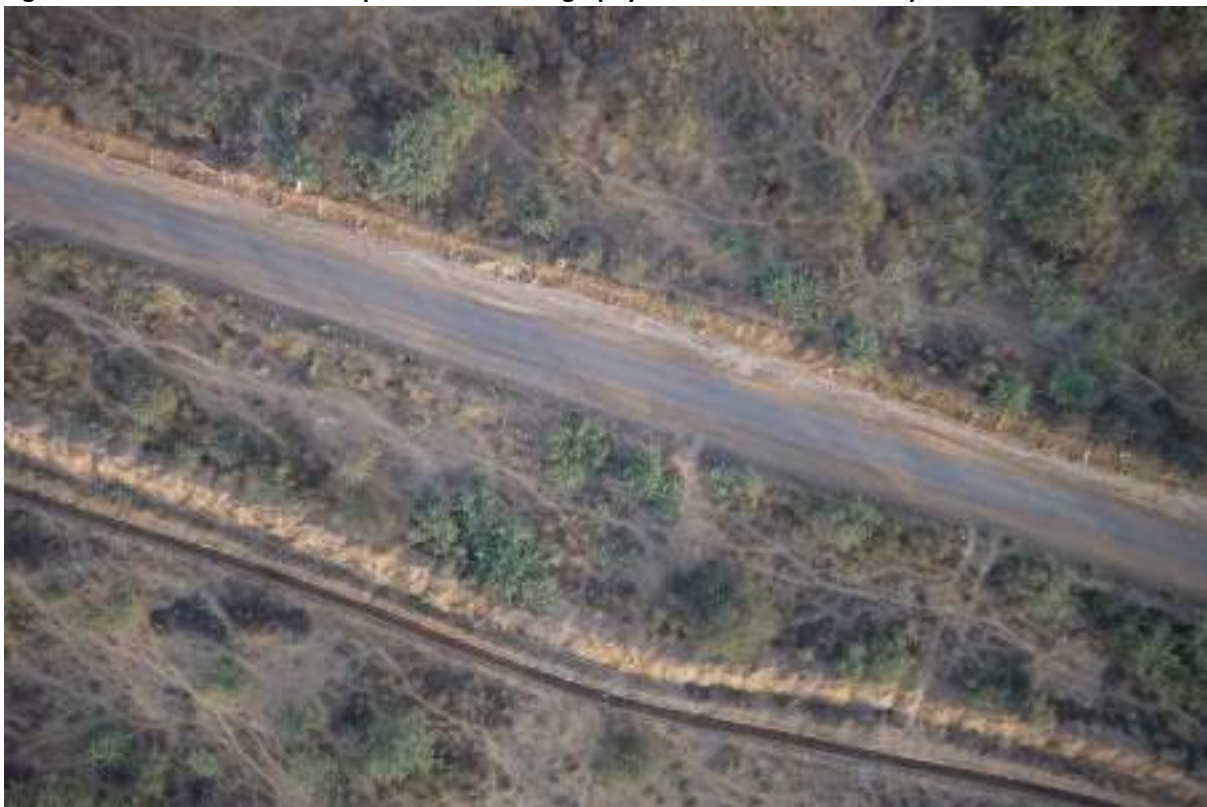
Fig 3.3.20 Aerial View of main / Asphalt road
