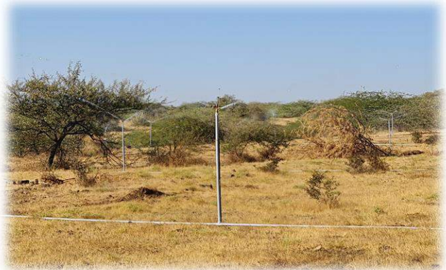
Fixed type water sprinkling system provided to check dust emissions at project
