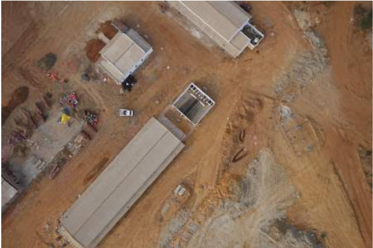
Fig 3.3.10 Aerial View of infrastructure
