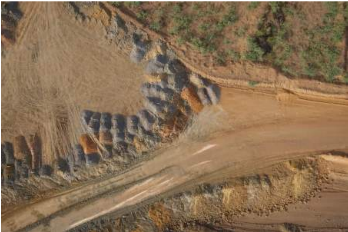
Fig 3.3.15 Aerial View of stack and waste Dump
