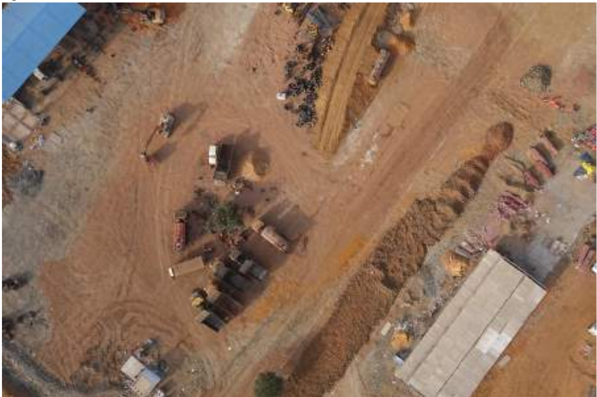
Fig 3.3.13 Aerial View of Contractor camp workshop
